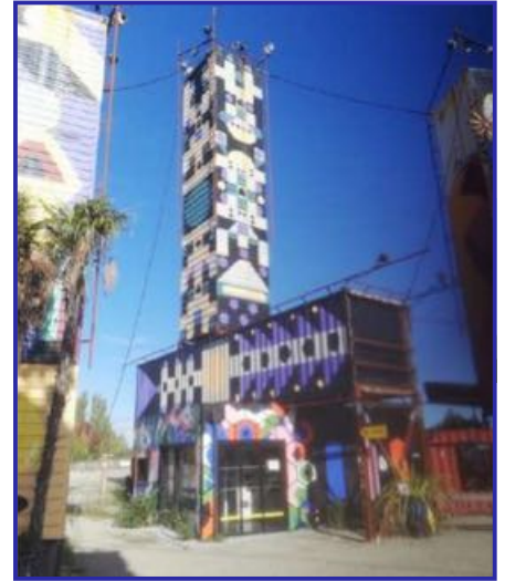
Point Info ( ossature bois + container)
